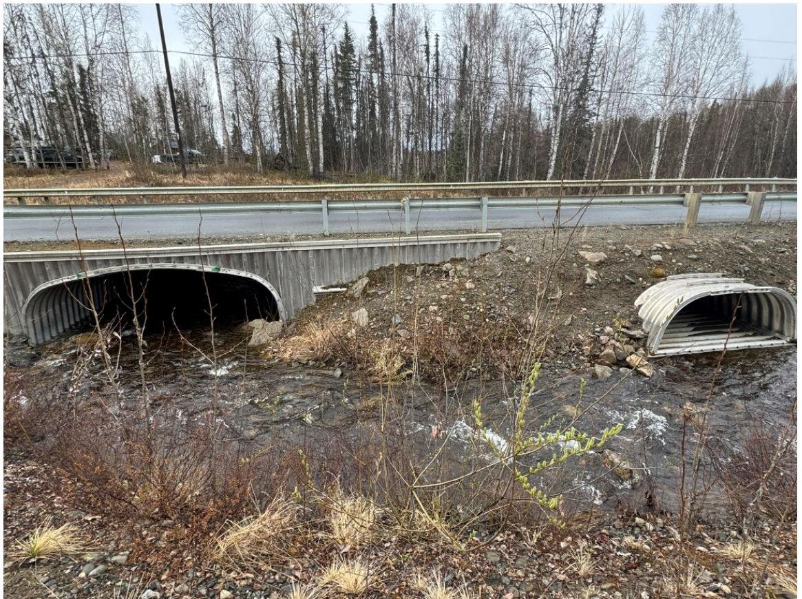
Figure 3-1. Upper Caswell Lake Outlet Culverts
