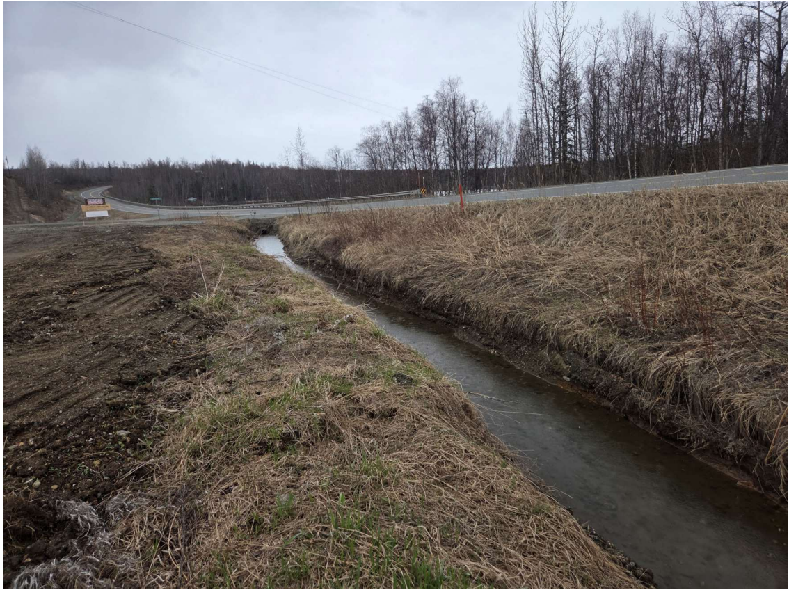
Figure 3-6. Knik Lake Outlet Channel – Upstream of Knik Bar & Grill Driveway
