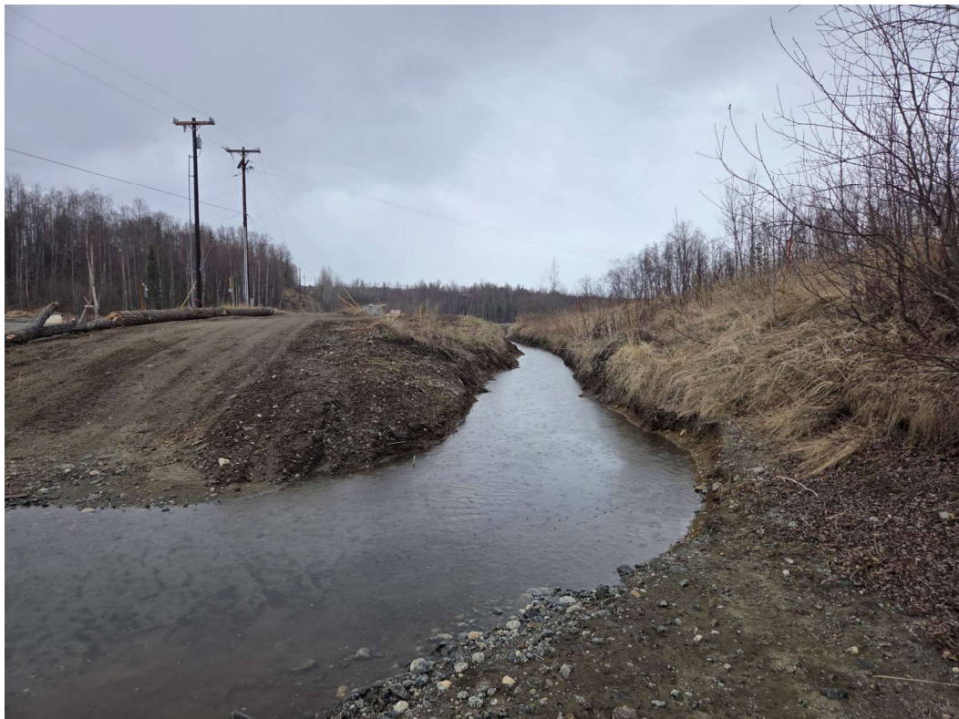
Figure 3-5. Knik Lake Outlet Channel - Looking Downstream
