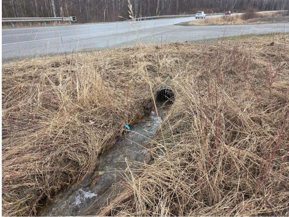
Knik Lake Outlet Culvert
