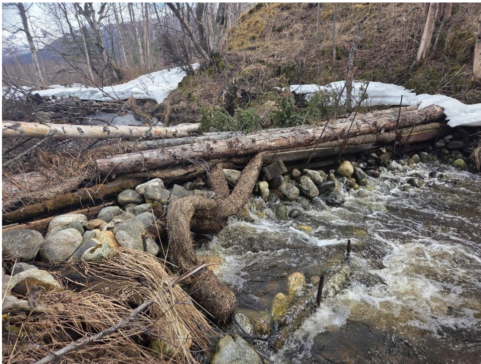
Wolverine Lake Outlet Structure
