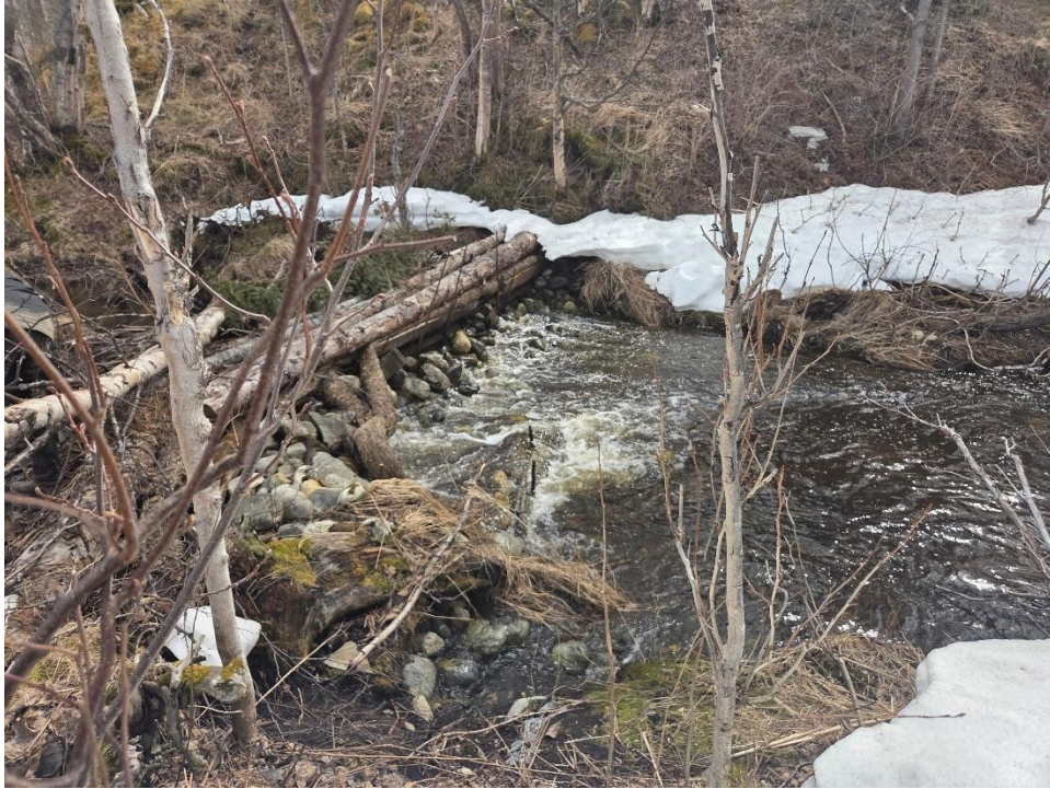
Wolverine Lake Outlet Structure
